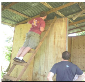
Carpenters at Work. Adam Nollsch on ladder, Brian Hurlbut.
